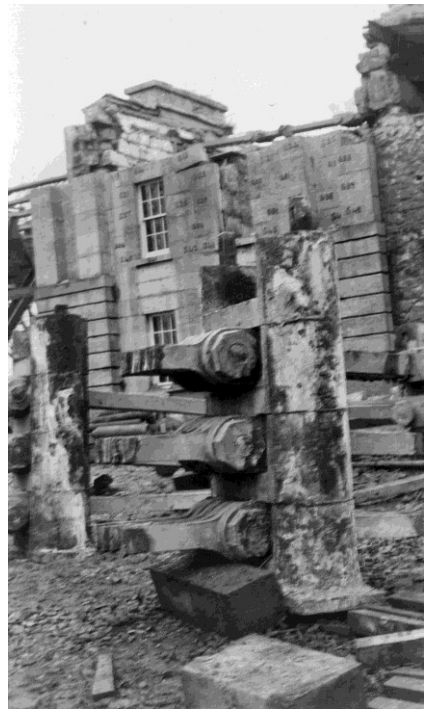
Figure 124 – View of intermediate saddles removed from Bridgmaster's House. (RE)
