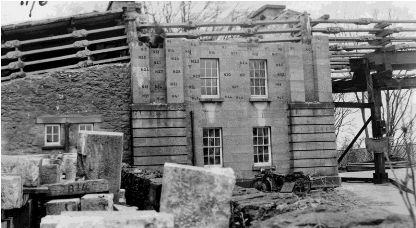
Figure 123 – Showing progress on the dismantling of the Bridgmaster's house. (RE)
