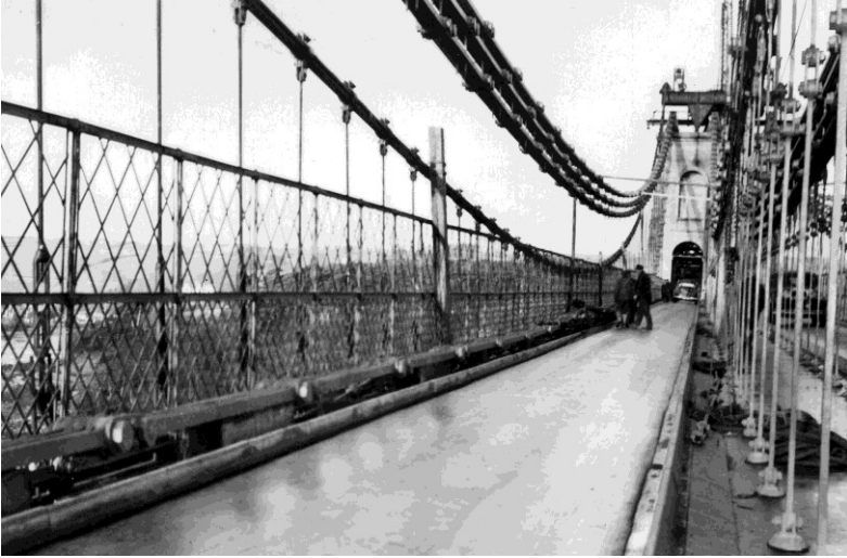
Figure 121 – Showing chain after lowering to deck. (RE)
